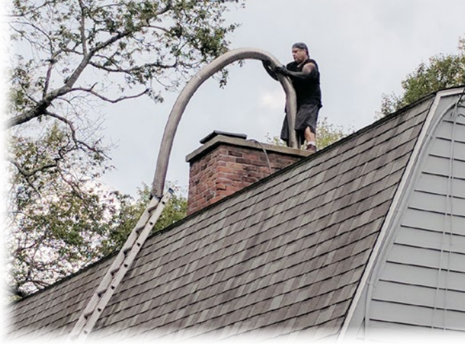
New chimney liner to boiler installed. 2017.
