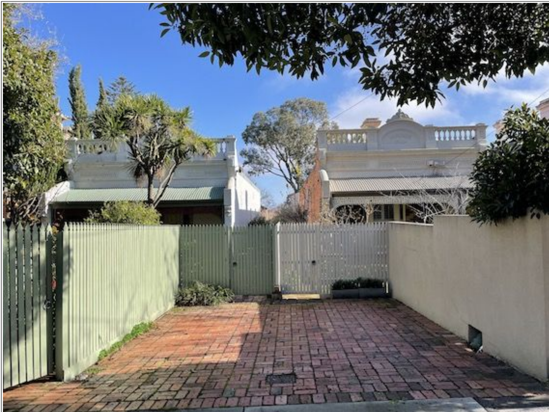
Number 32 (ours) on the left and number 30 on the right; with shared off-street parking area.
